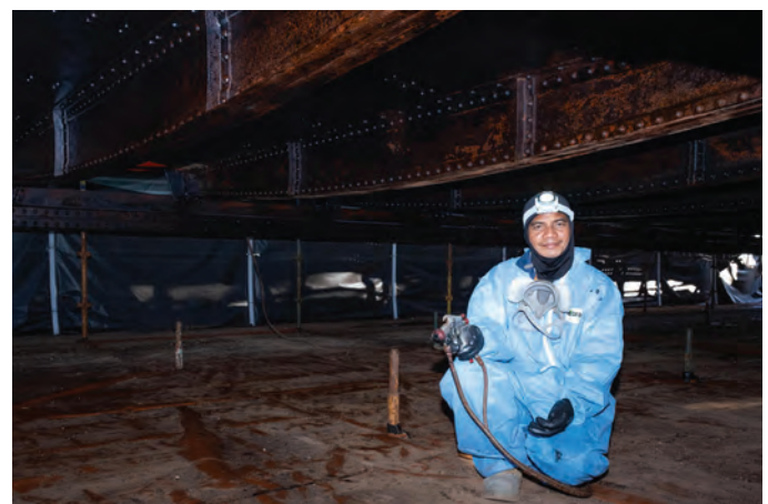
Work on Dunn's Bridge to renew the historic 143-year-old structure.
