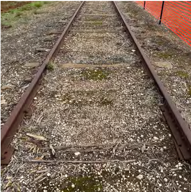
railway track - infill between track with compacted fines or similar creating safe flat walkway and featuring the railway heritage
