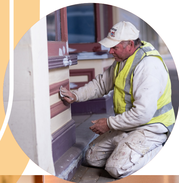
ABOVE: Wayne Treverton working on façade improvements in Balaklava
