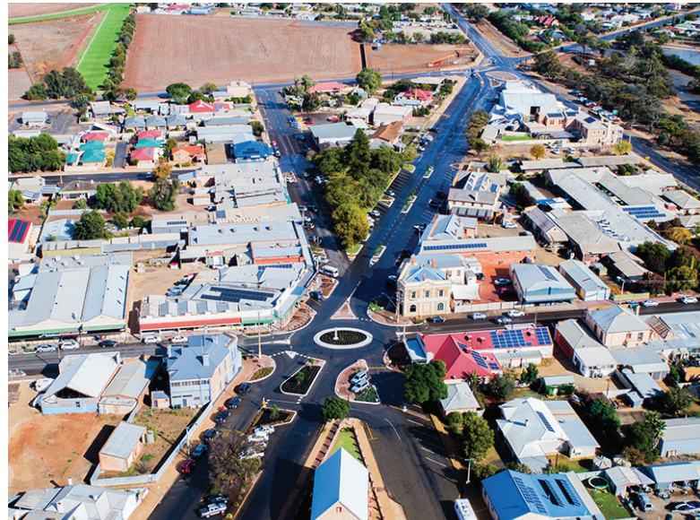
An aerial view of the completed Balaklava Main Street upgrade.
