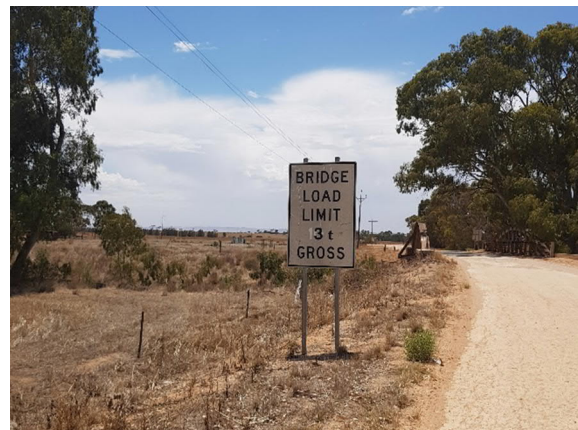
Image 2 BR006 Dunns Bridge (3T)
