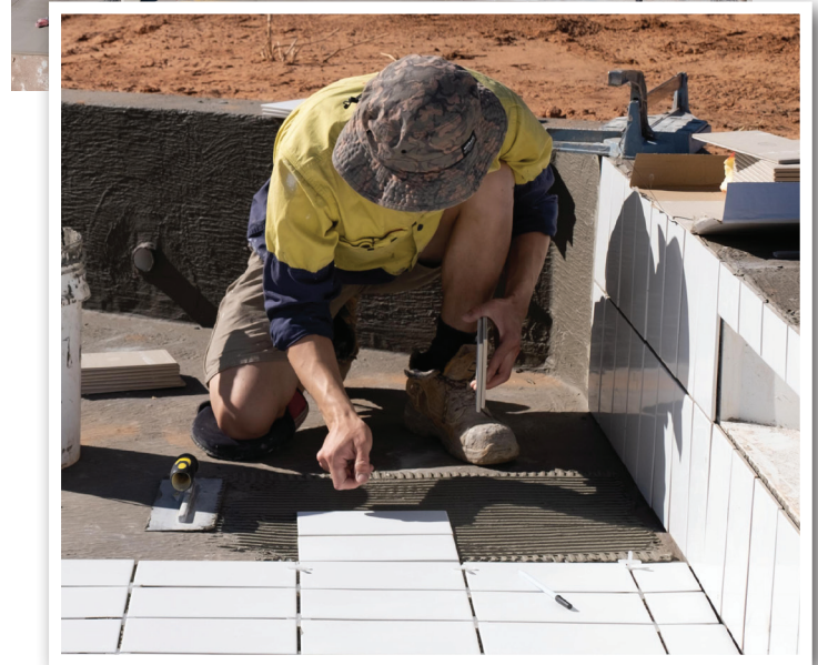
ABOVE: Tiling the wading pool at Owen. TOP: The beginning of the 25m pool's tiling.
