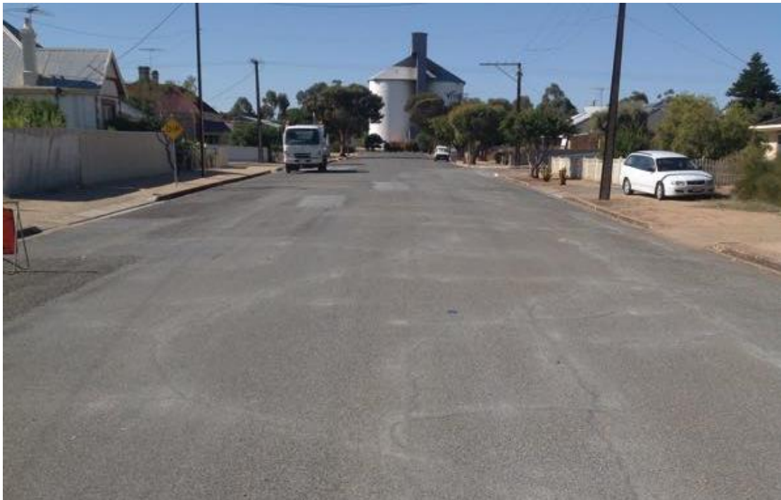
Typical Township Sealed Road with preparation works prior to seal, which can be applied as a proactive maintenance activity
