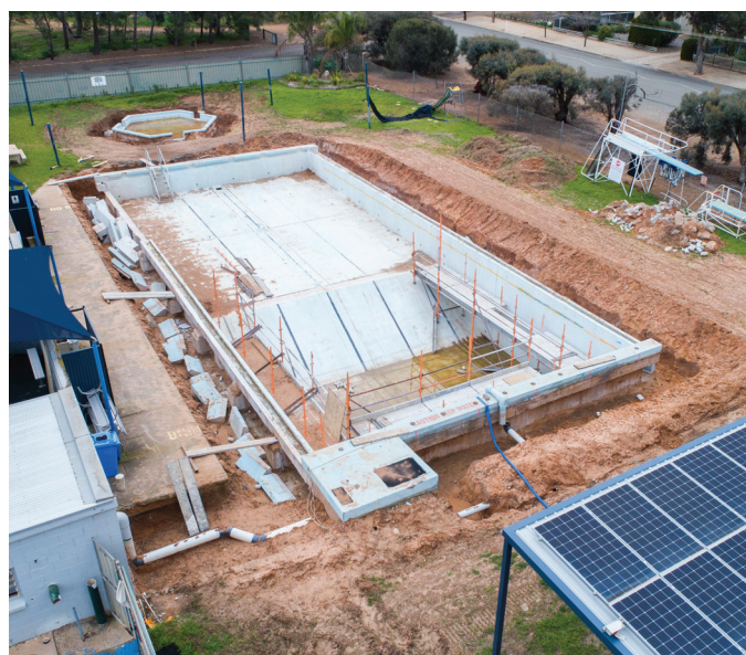
The Owen Swimming Pool works are well on their way.
