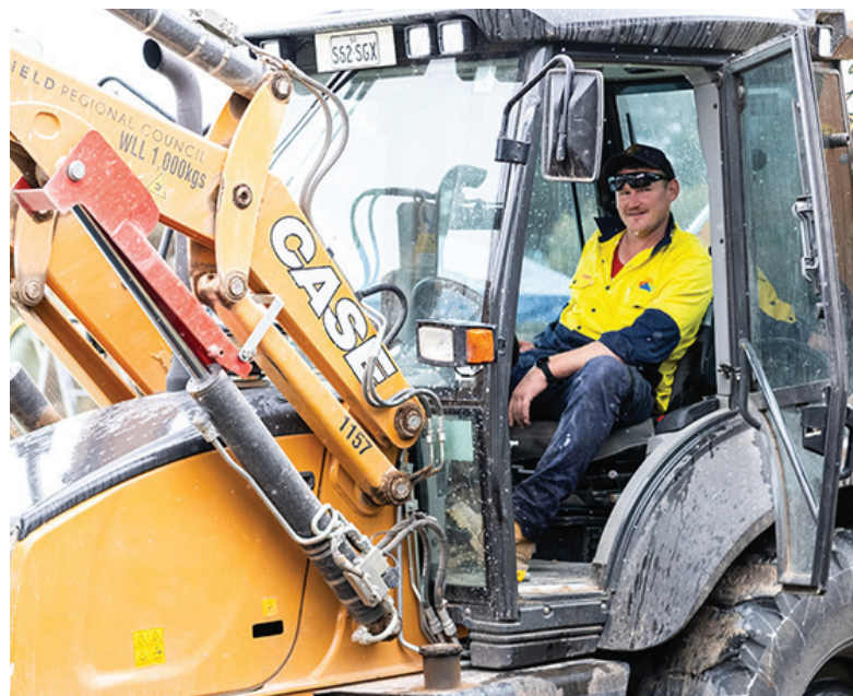
Works crew member Jamie Williams onsite at the Owen Swimming Pool.
