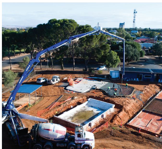
Splashpad construction at the Balaklava Swimming Pool in May 2022.
